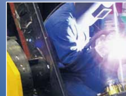
SEMI-AUTOMATIC WELDING of CW jump pipes
